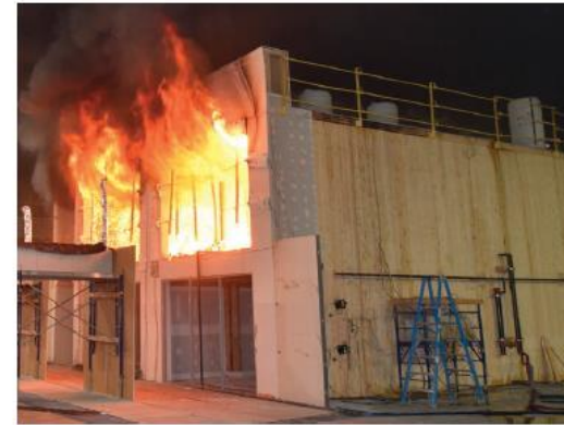
Figure 7-3 The TWB-AHC determined fire testing was necessary to validate established performance objectives. Consequently five, full-scale, multiple-story fire tests were conducted to simulate the three new construction types (Types IV-A, IV-B and IV-C).
