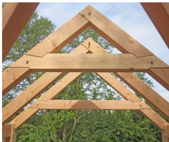
Figure 13 • Traditional Roof Trusses
