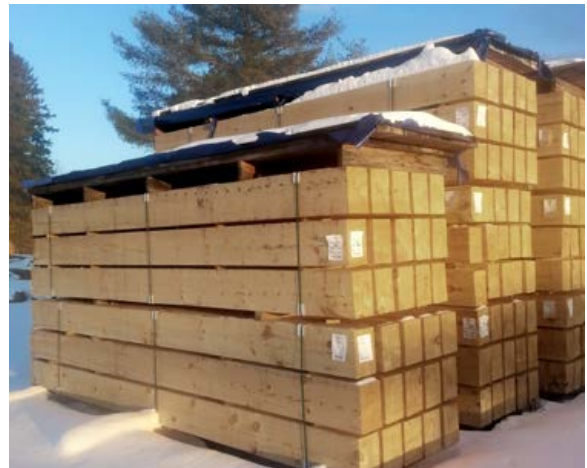
Figure 7 - Well Stickered and Bundled Heavy Timber components
