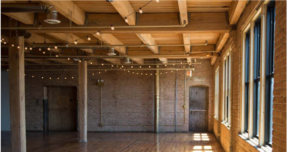
Figure 10 • Traditional Posts and Beams System
