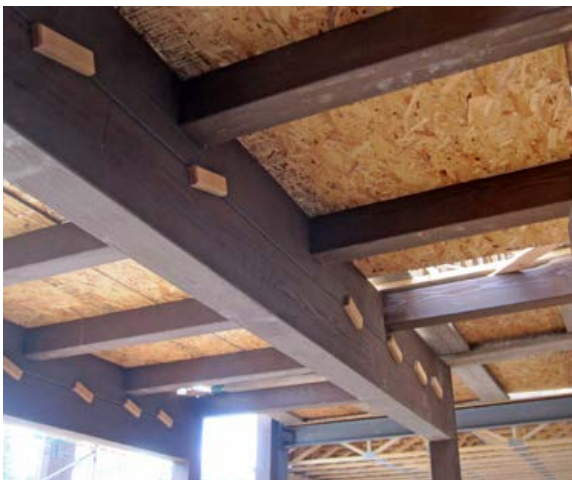
Figure 14 • Key Beam Girders
