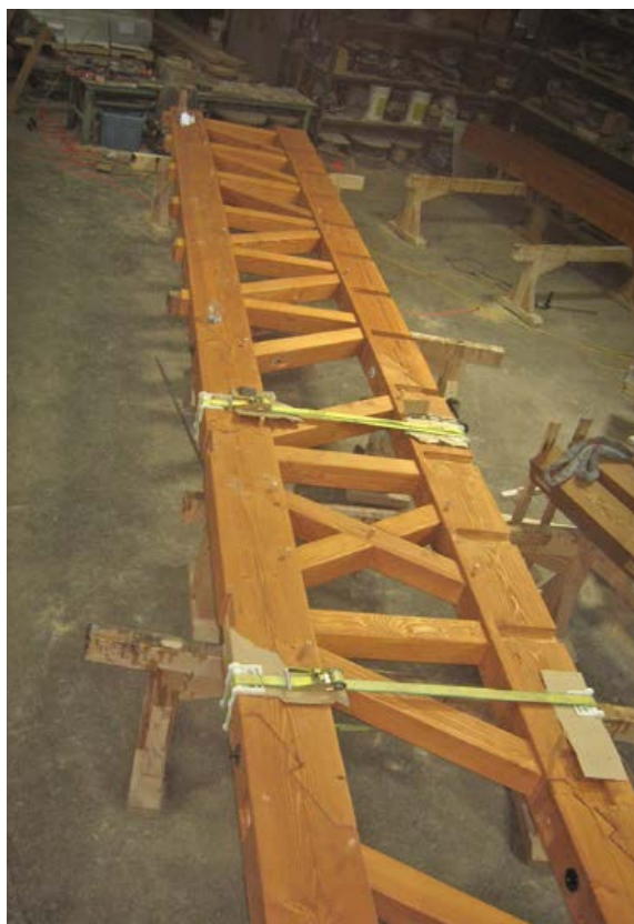
Figure 12 • Fabrication of a Timber Flat Roof Truss
