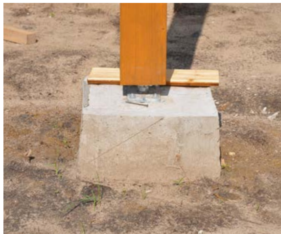
Figure 18 • Good Post Base Design
